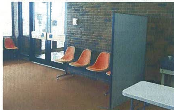
The wall between the Holdroom and Baggage Make-up Room will be relocated.
