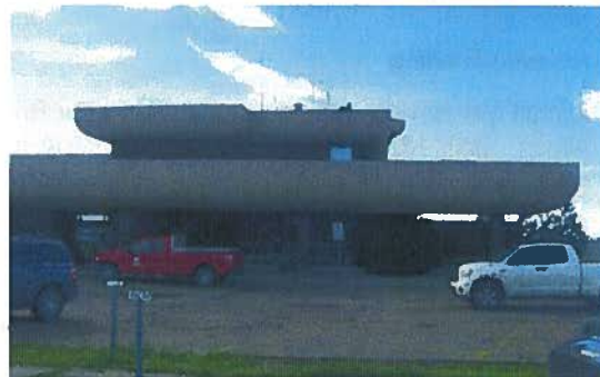
The Terminal Frontage Road has recently been rehabilitated.
