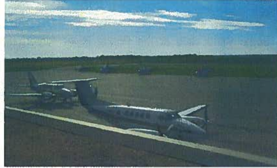
Apron I can provide four (4) aircraft stands accommodating the B737-400, DHC8-400, B1900D, and B350 aircraft.
