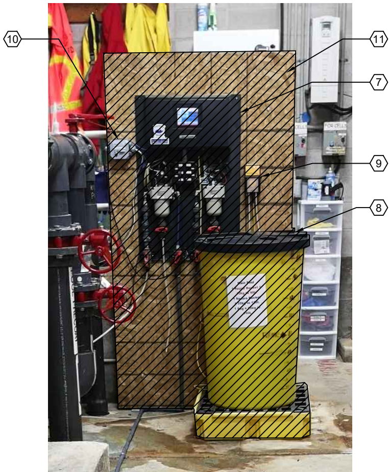
3 MAIN POOL ACID FEED RELOCATION SCALE: NTS
