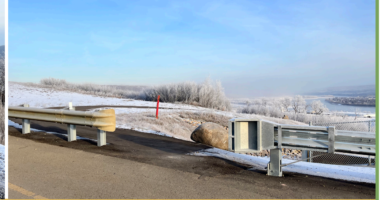
View to Northeast at Trail Access/ Old Hwy 2 off-ramp
