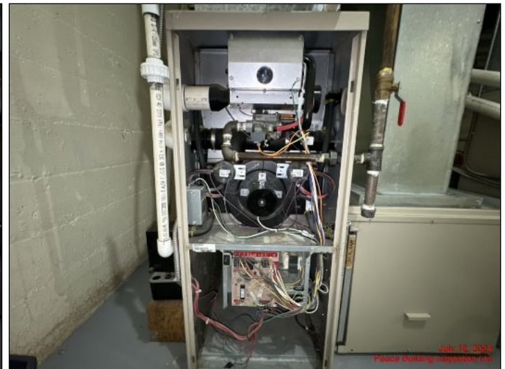
All furnace interiors in good condition at time of inspection
