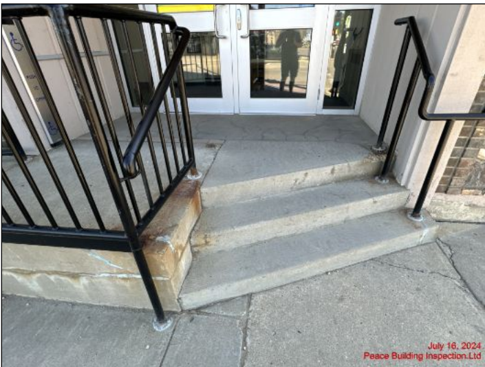
Concrete front steps in good overall condition at time of inspection
