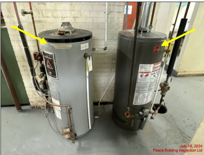
Building equipped with a solar water heater and a conventional water heater
