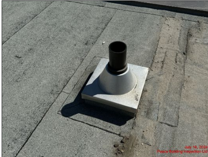
Plumbing vents in good condition at time of inspection
