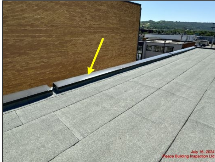
Roof parapet edge flashing in good condition at time of inspection
