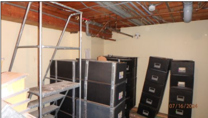
Storage area in good condition at time of inspection
