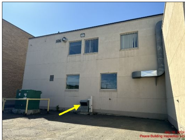
Combustion air in good condition at time of inspection
