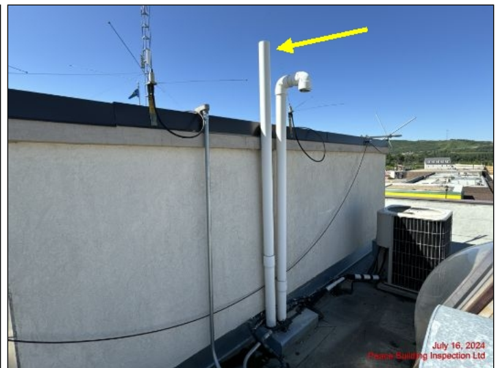
Upper furnace exhaust vent in good condition at time of inspection
