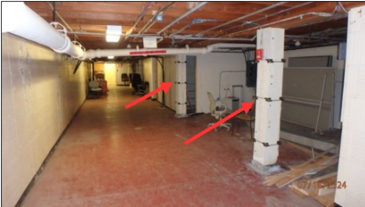
Building equipped with wood support posts
