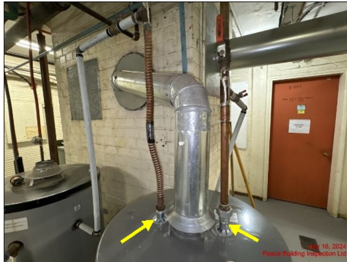
Water heater pipe connections in good condition at time of inspection
