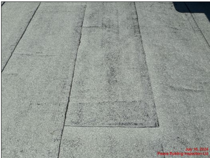
Roof cover in good condition at time of inspection
