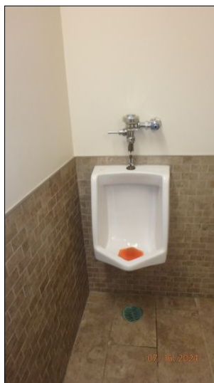
Mens urinals in good condition at time of inspection
