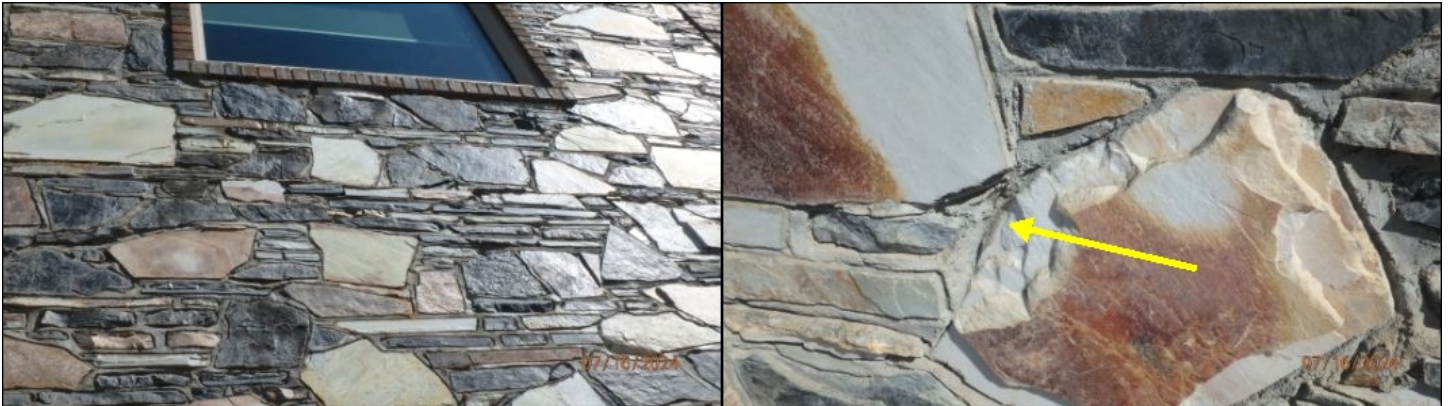
Stone exterior walls in good condition at time of inspection
