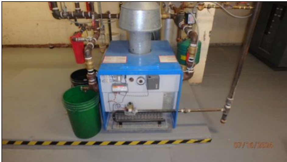
Boiler in good condition at time of inspection
