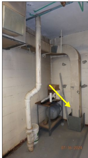
Boiler room combustion air in good condition at time of inspection
