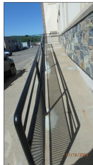
Side exterior ramp in good condition at time of inspection
