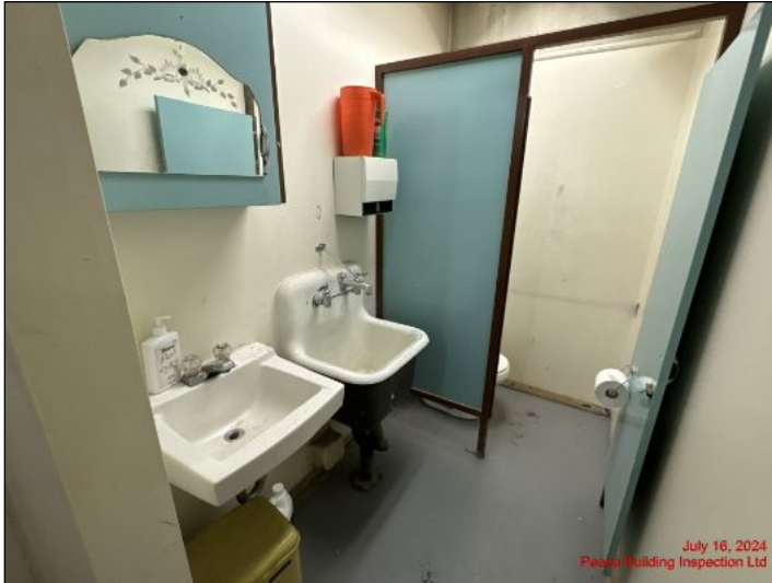
Basement bathroom in good condition at time of inspection
