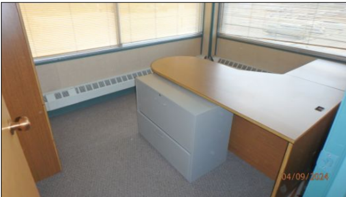
Most interior rooms in acceptable condition at time of inspection
