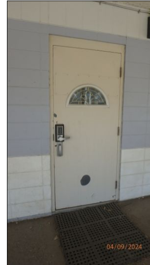
Rear exterior door in good condition at time of inspection
