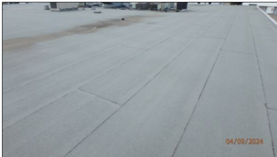
Roof cover in good condition at time of inspection
