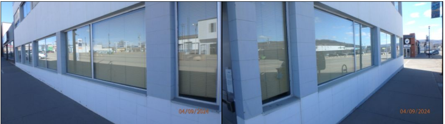
Exterior windows in mostly good condition at time of inspection
