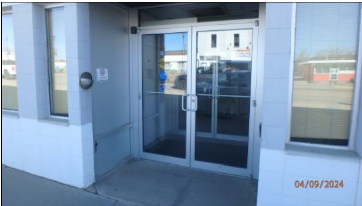
Front doors in good condition at time of inspection
