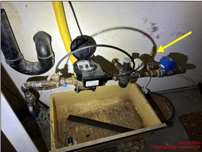
Main water supply line was shut off at time of inspection
