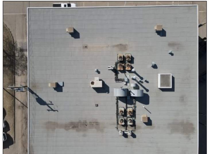
Roof also examined with a drone
