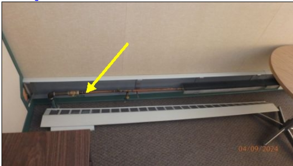
Repair any baseboard radiant heater covers that are damaged or missing
