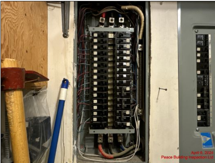
All service panel interiors in mostly good condition
