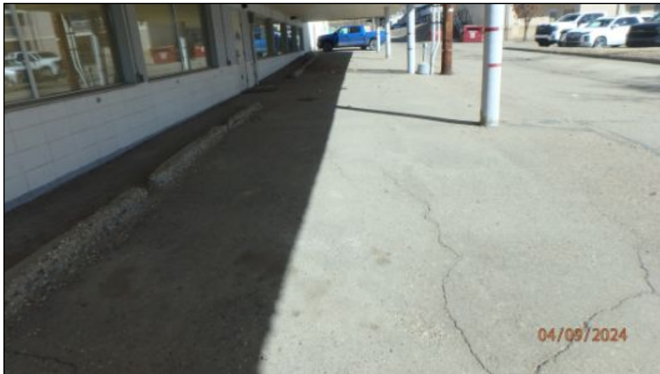
Asphalt driveway/parking lot in good condition at time of inspection
