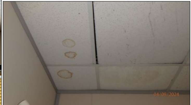
Upper level ceiling stains were dry at time of inspection
