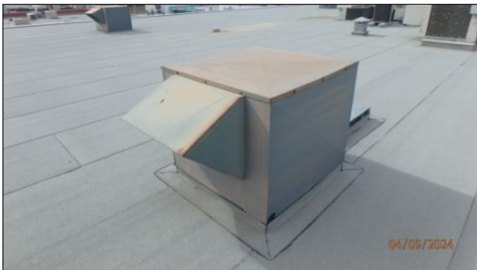
Roof vents in good condition at time of inspection
