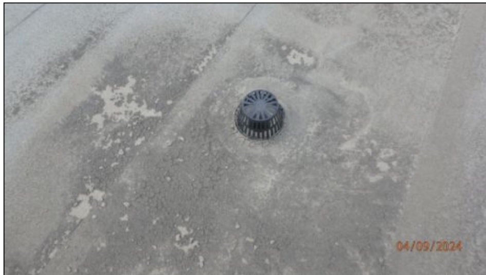
In roof drains in good condition at time of inspection
