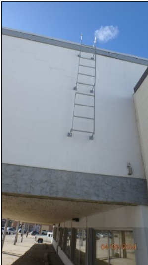
Roof was accessed via this ladder
