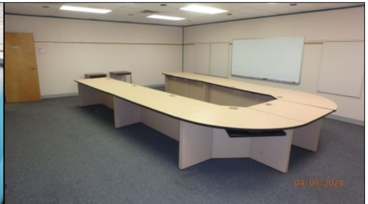
Most interior rooms in acceptable condition at time of inspection
