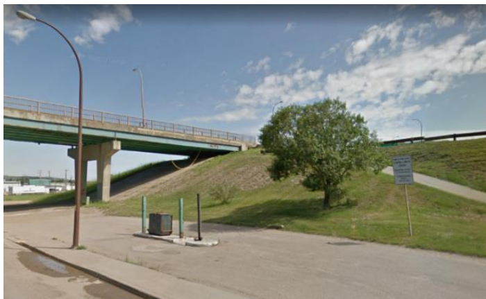
Sanitary Sewer Transfer Station
