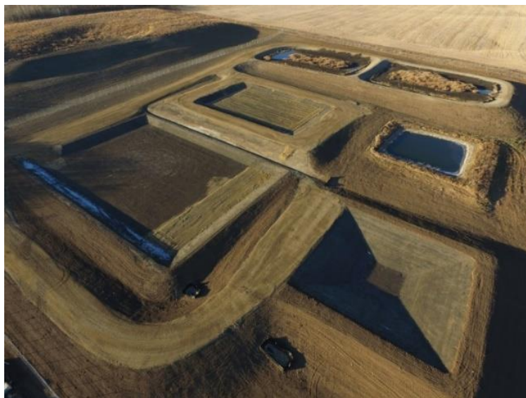
Weberville Drying Beds and Leachate Ponds
