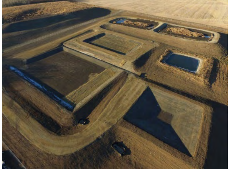
Weberville Drying Beds and Leachate Ponds
