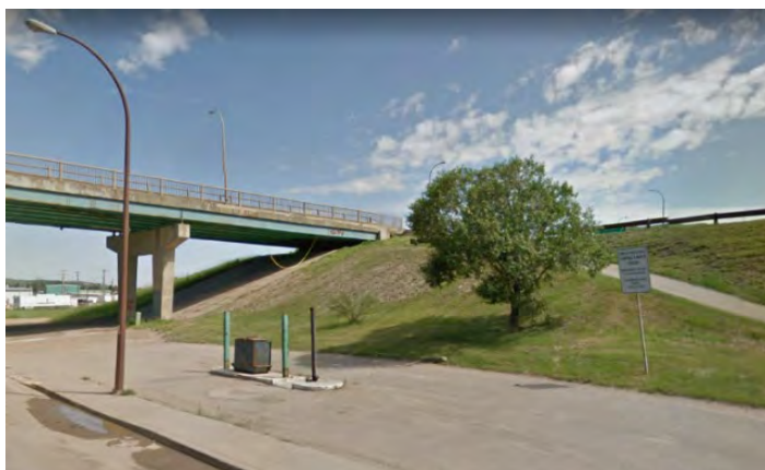
Sanitary Sewer Transfer Station
